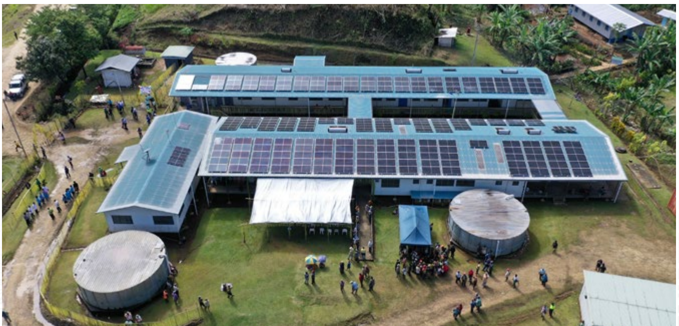
Pimaga Rural Hospital solar mini grid project funded by Santos Foundation and the US-AID Papua New Guinea Electrification Partnership. (Pic supplied by Santos).
