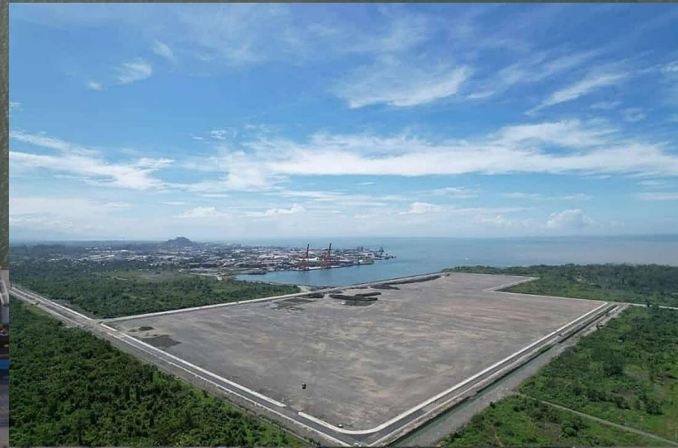
Phase 2 of the Lae Tidal Basin
