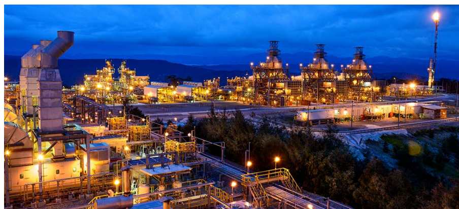
The Hides Gas Conditioning Plant
